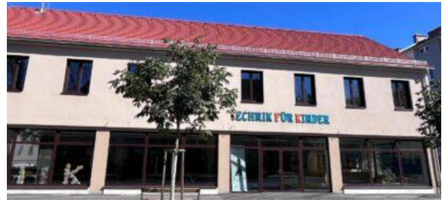
Fig. 2. Exterior View of the Technology House
